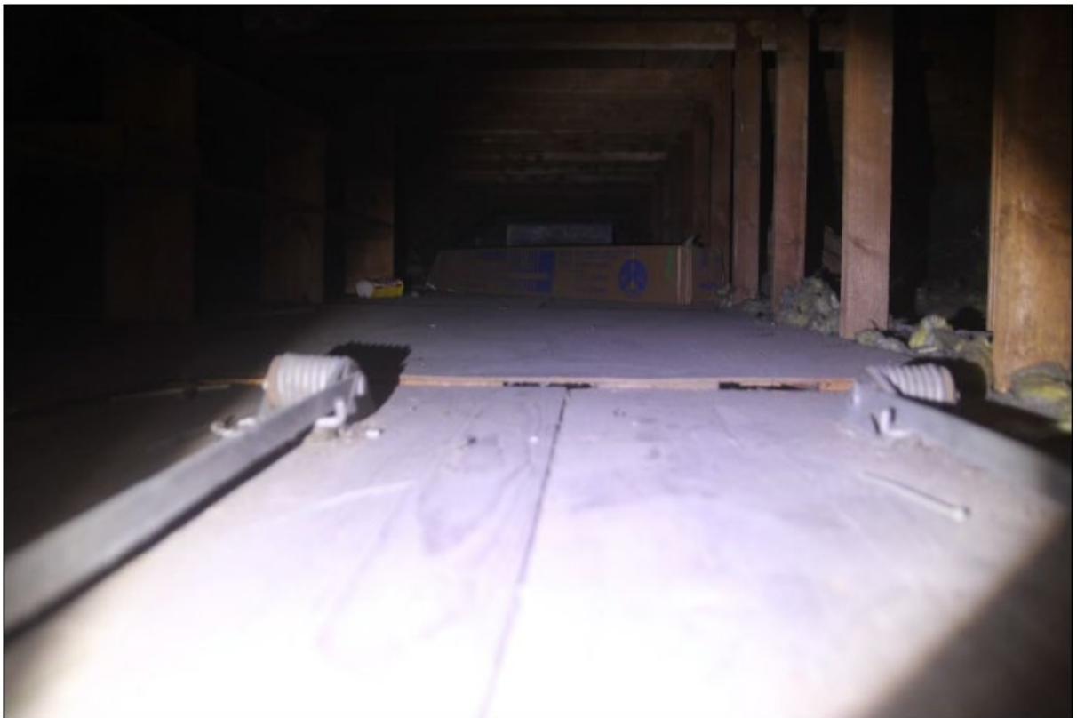
Plate 2 Attic space of Building 17 reveals no signs of bats – inspected March 1 st 2022
