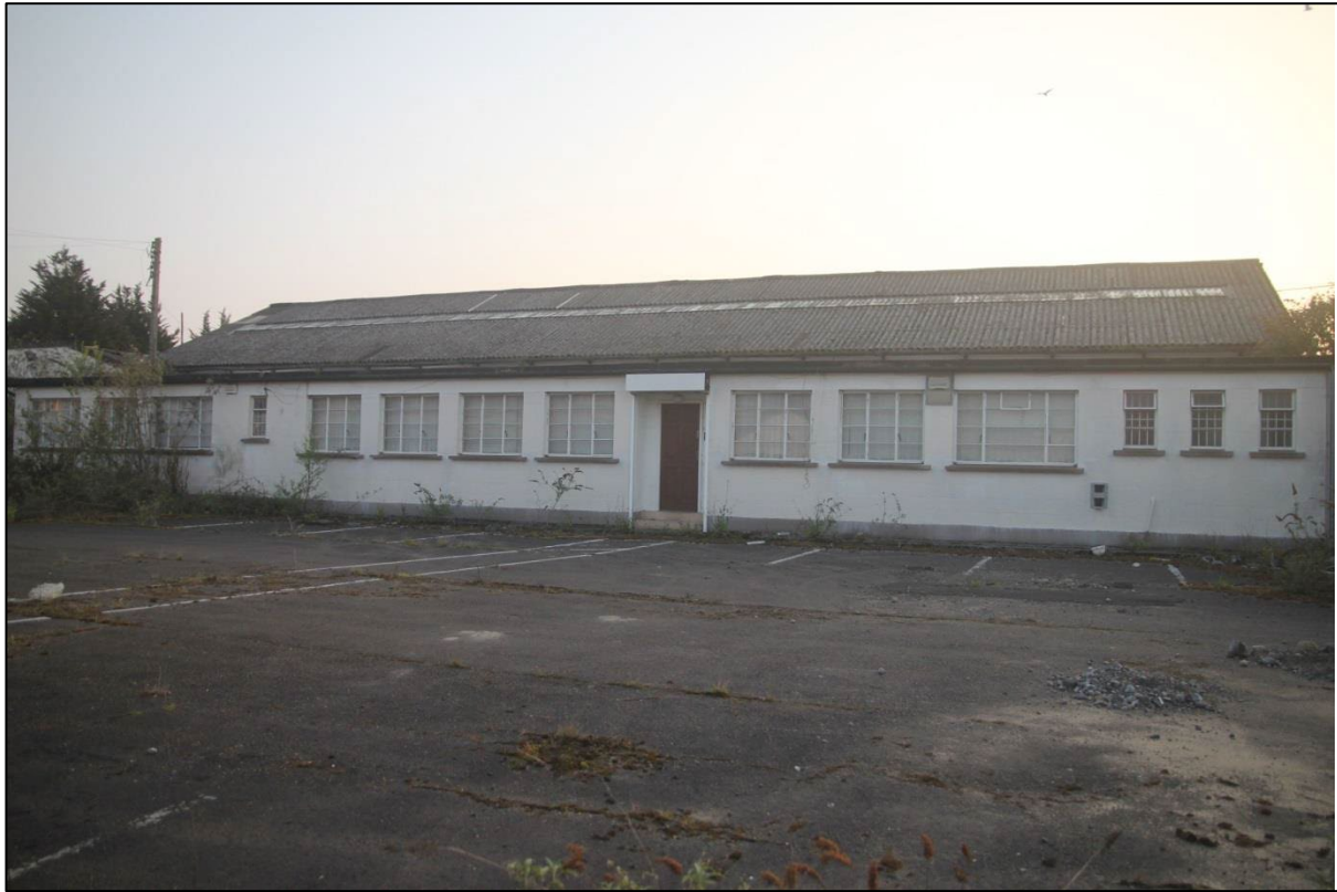
Plate 9 Building 9 – Low Bat Potential.
