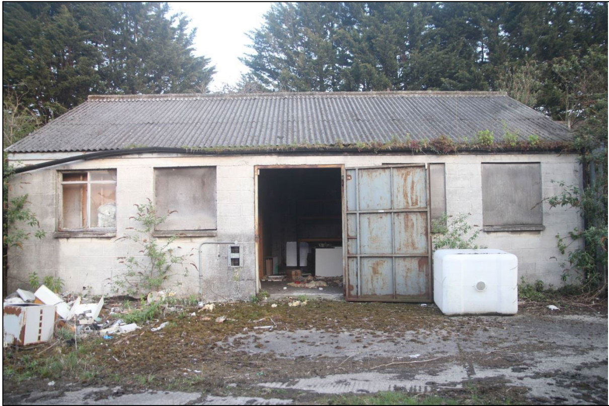
Plate 7 Building 7 - Low Bat Potential.
