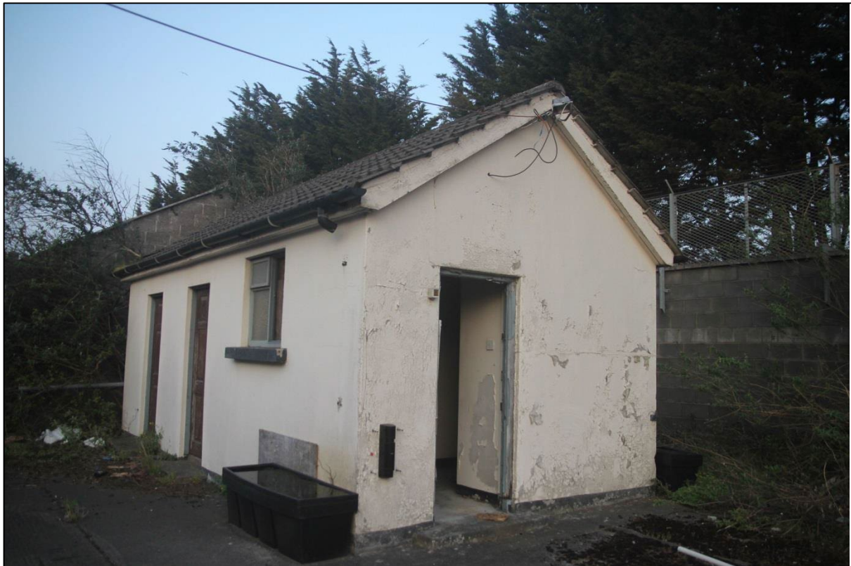
Plate 8 Building 8 - Low Bat Potential.
