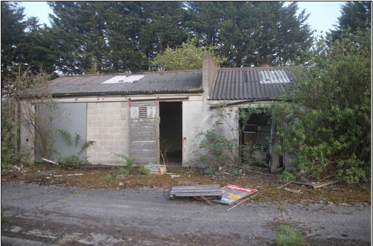
Plate 6 Building 6 - Low Bat Potential.
